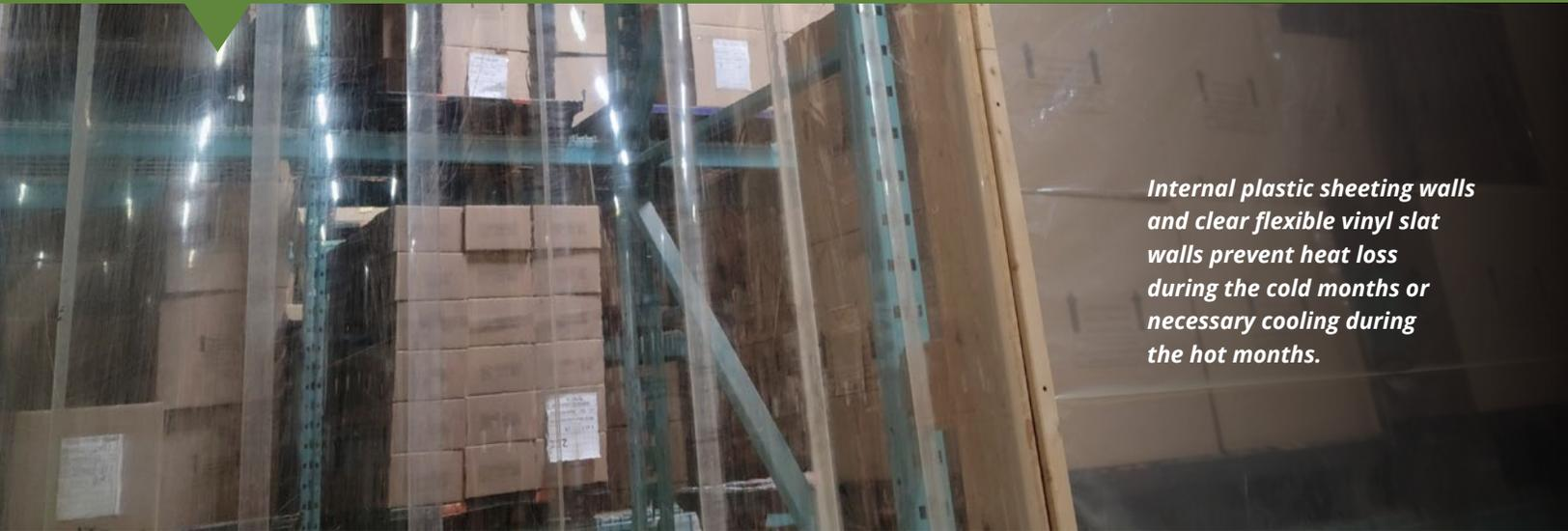
*Internal plastic sheeting walls and clear flexible vinyl slat walls prevent heat loss during the cold months or necessary cooling during the hot months.*
