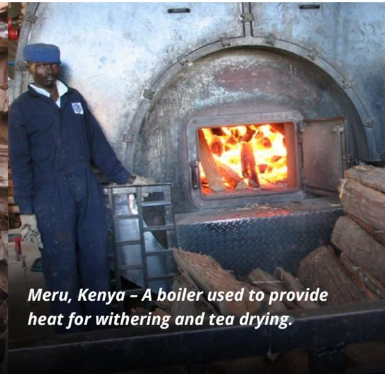
*Meru, Kenya – A boiler used to provide heat for withering and tea drying.*
