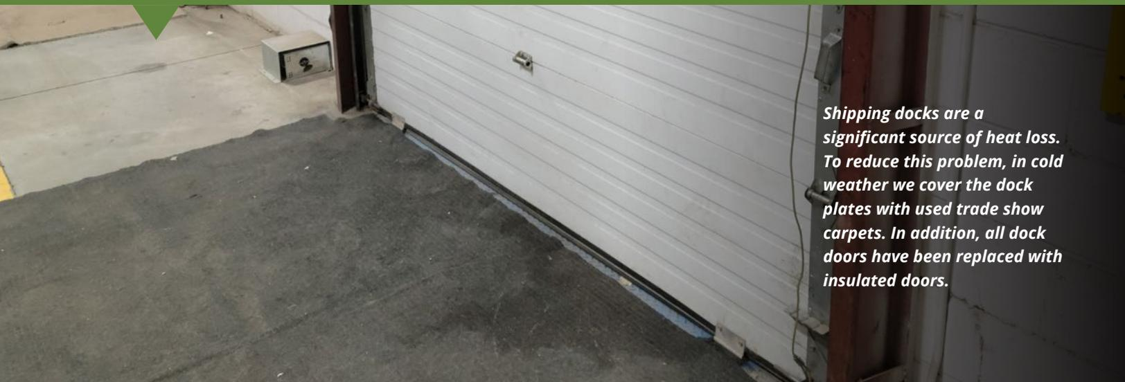
*Shipping docks are a significant source of heat loss. To reduce this problem, in cold weather we cover the dock plates with used trade show carpets. In addition, all dock doors have been replaced with insulated doors.*
